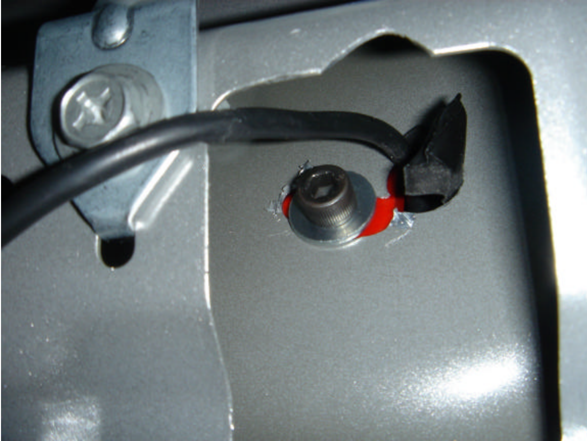
Photo 12 – cable entry for camera
